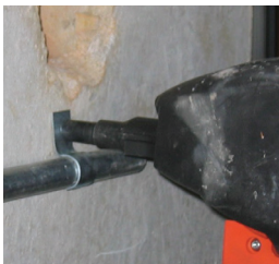
12HSMP034 clip assembly used to secure conduit
