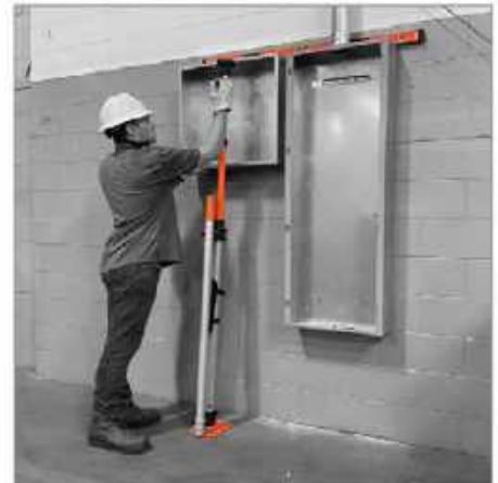
One handed gas shock operation
